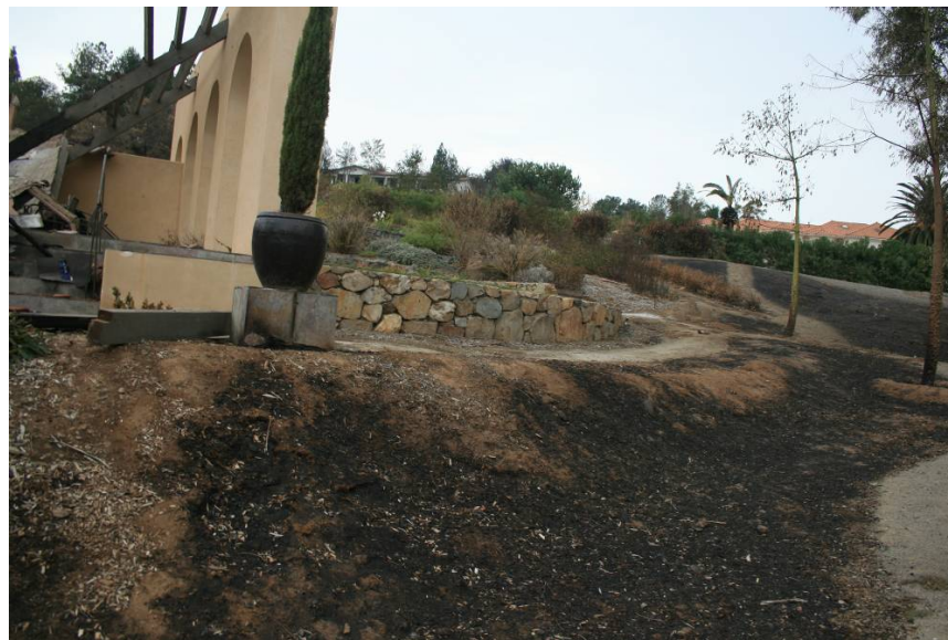
Figure 27: Structure Ignition Category B
