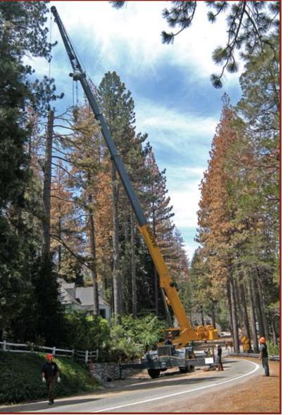
**Figure 20.** Large dead tree removal on private property. These dead trees posed a risk of falling on roadways, homes, power lines, and other structures. In addition, once ignited they cast embers to ignite spot fires in wildland fuel and structures. Removal of these trees lessened the risk to firefighters working in and around the structures.
