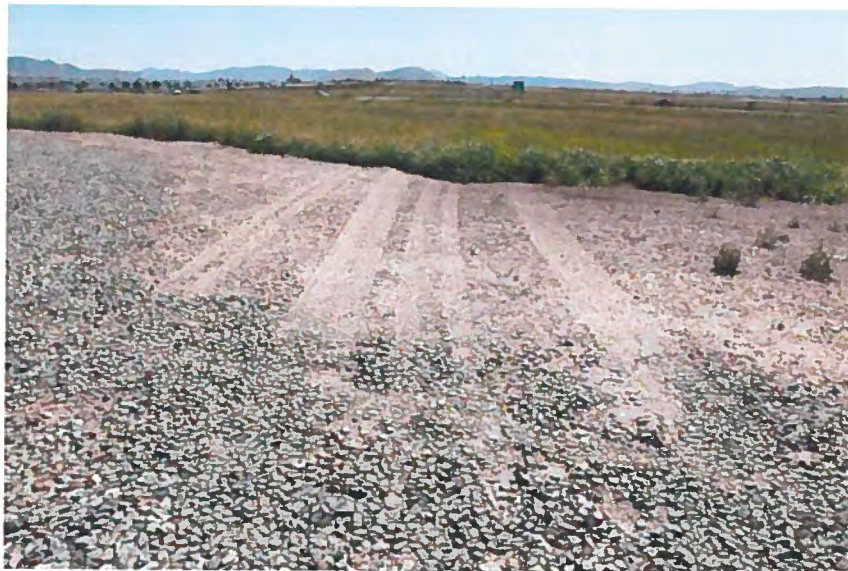
Tire Tracks Leading To Helicopter Pads South View from South Pad 3-3-2012
